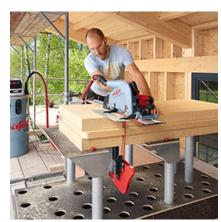
Whether you're cutting longways, crossways or at an angle, the plug-in supporting system for pressure-resistant and flexible insulating materials can be configured to suit any situation. Even when working on scaffolding.
