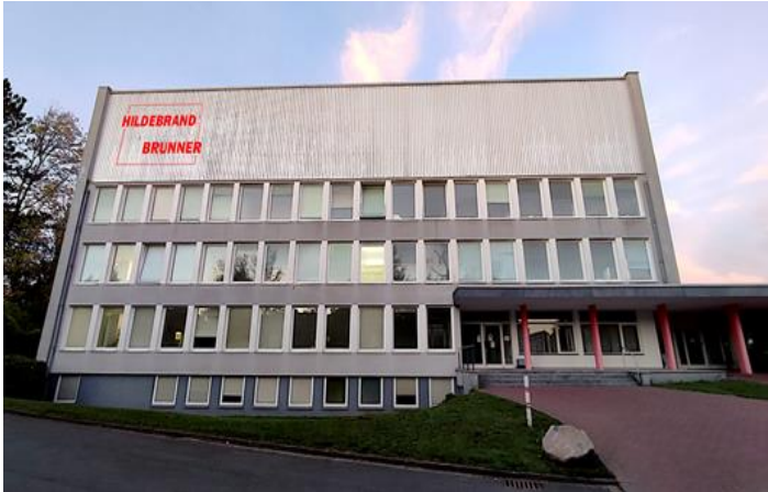
Headquarter Gehrden/Hanover - Germany
