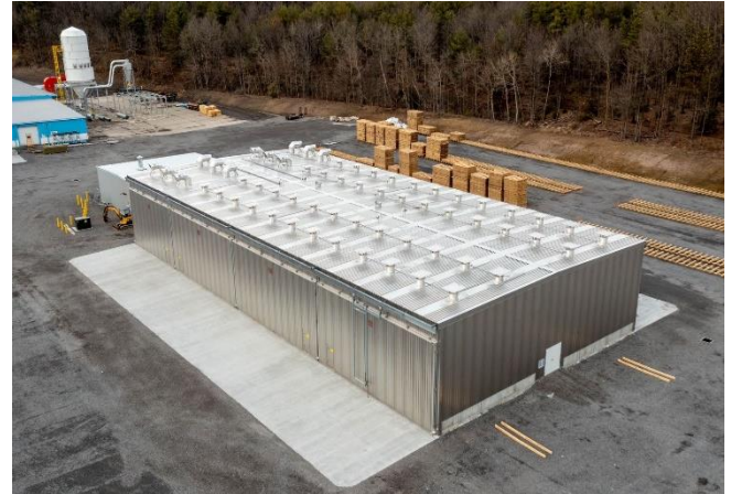
Project in Pennsylvania, USA 2022
